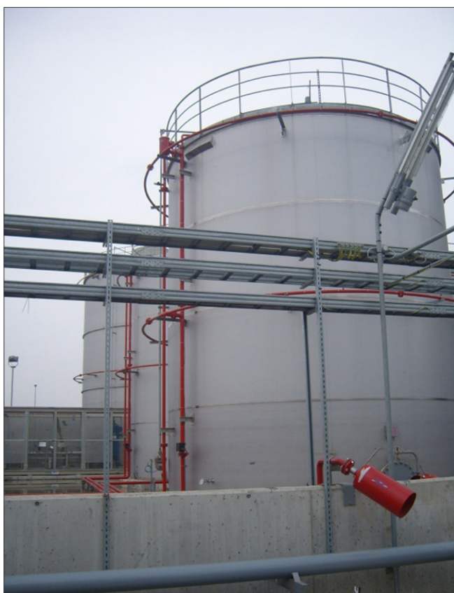
Fig. 2 - Fixed surface system and sprinklers
